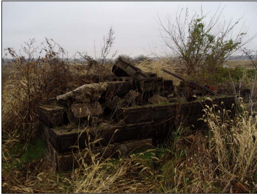
Photograph 7: Concrete block and stone debris from building.
