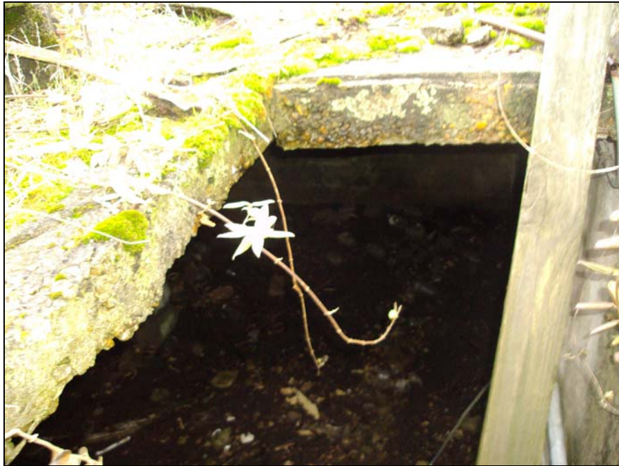
Photograph 8: View into basement of building remnants.
