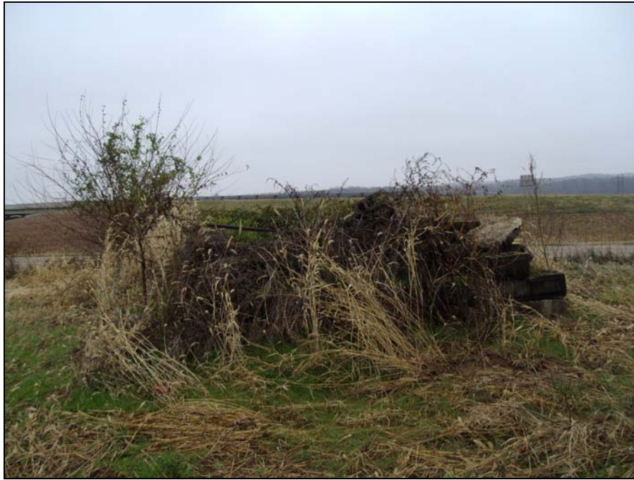
Photograph 3: Remnants of building.
